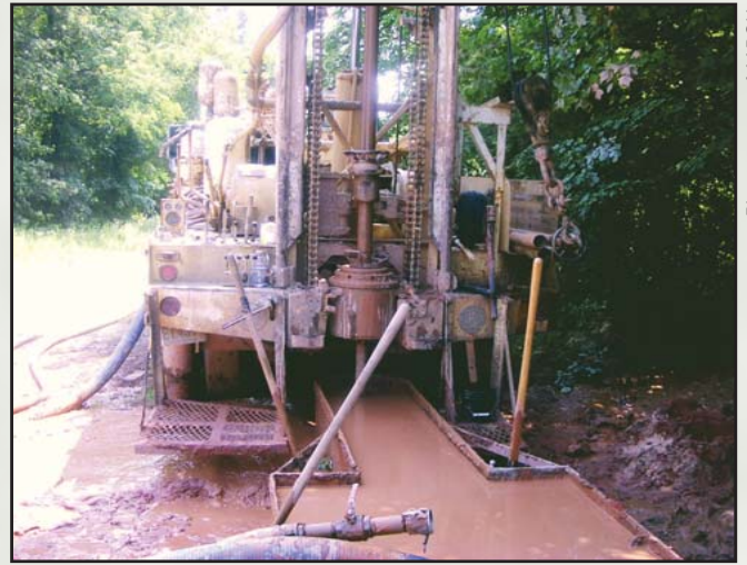
Figure 5. Drilling new, deeper residential well.
